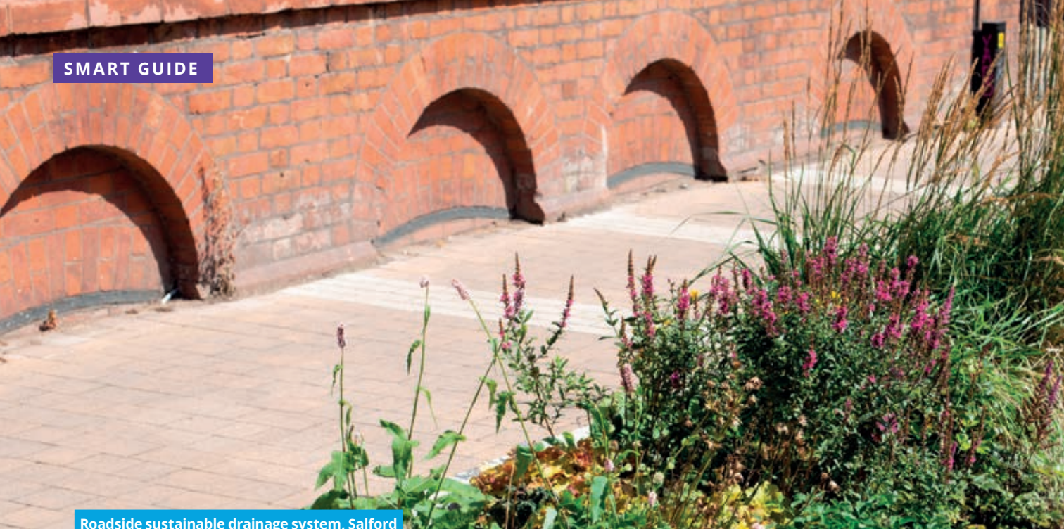
Roadside sustainable drainage system, Salford
